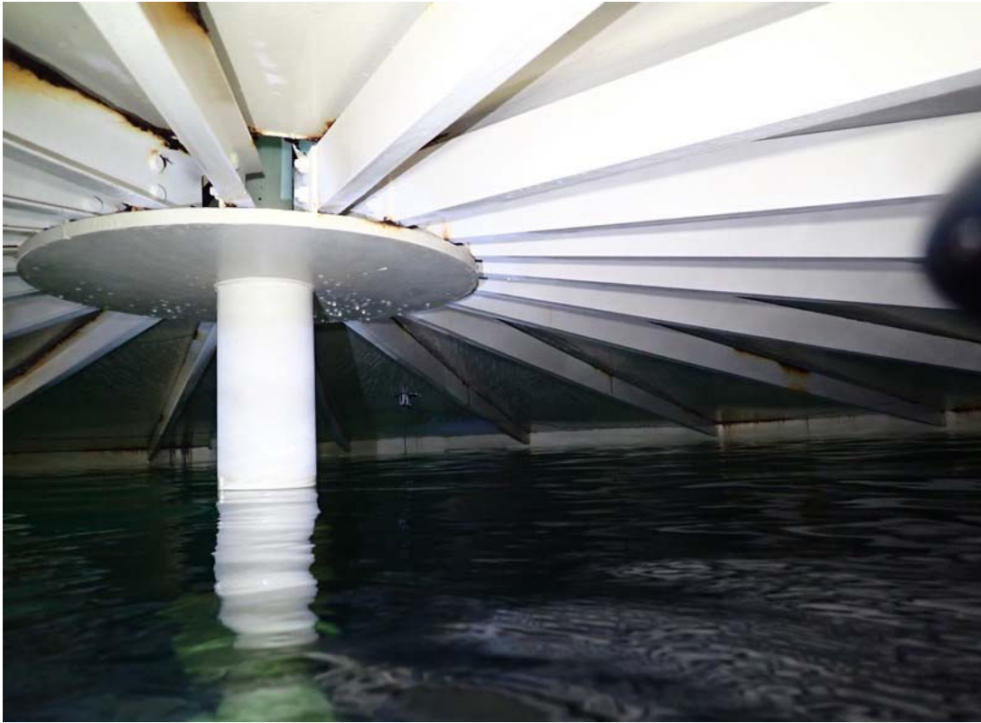
Upper center column, rafters and roof plate.
