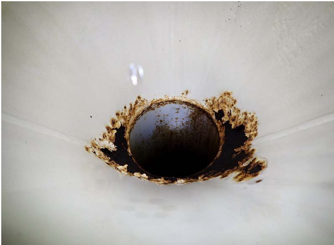
This view is of the inside of the overflow weir. Some corrosion is visible but the pipe appears to be free of obstructions.
