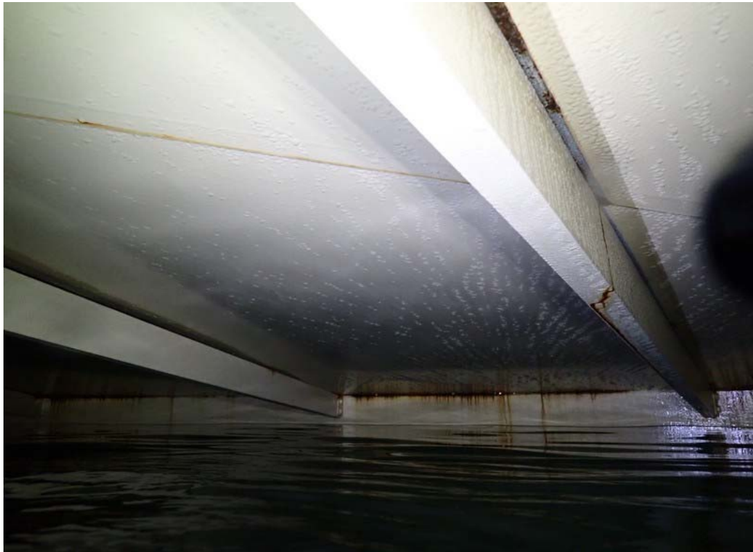
An additional view of the interior roof.
