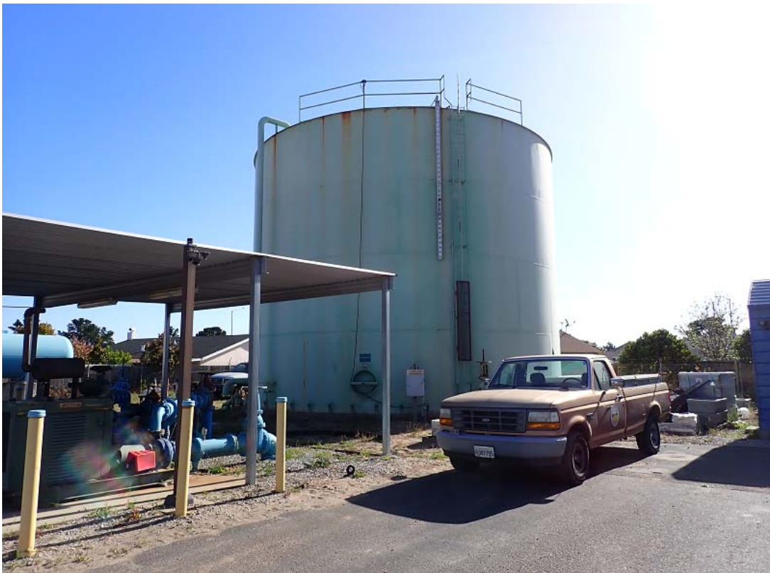
View of tank and portion of Contractor "lay-down" area.
