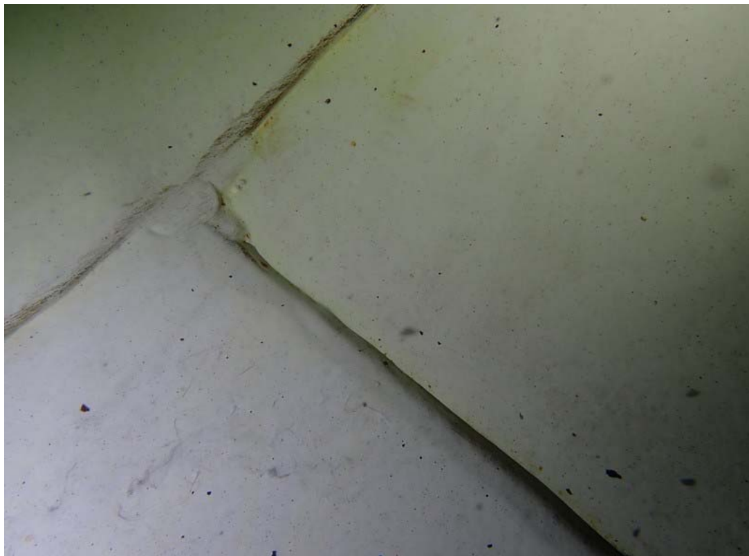
Close view of a weld in the bottom.
