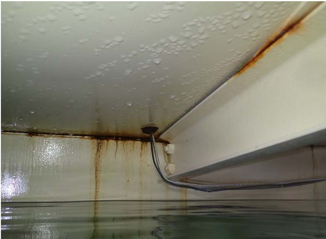
This view is representative of the conditions found on the interior shell, roof plate and rafter.
