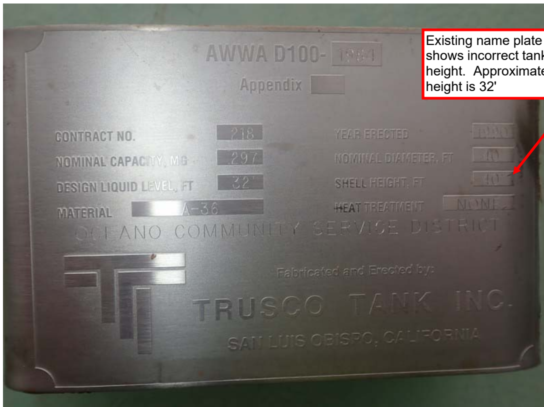
Original name plate with incorrect height shown.
