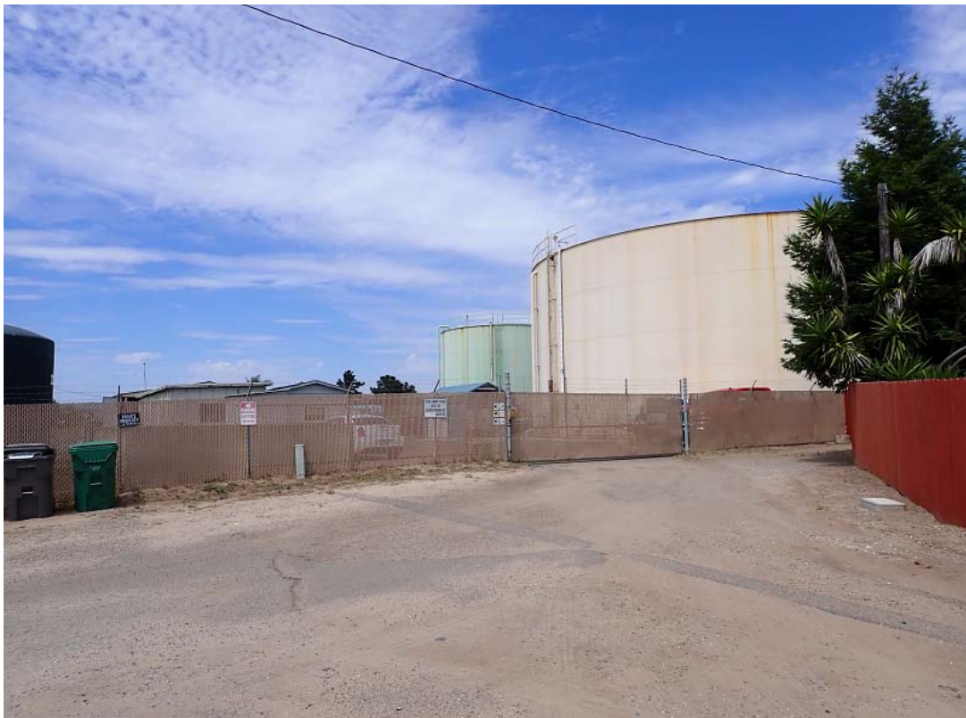
Access gate and tank site.
