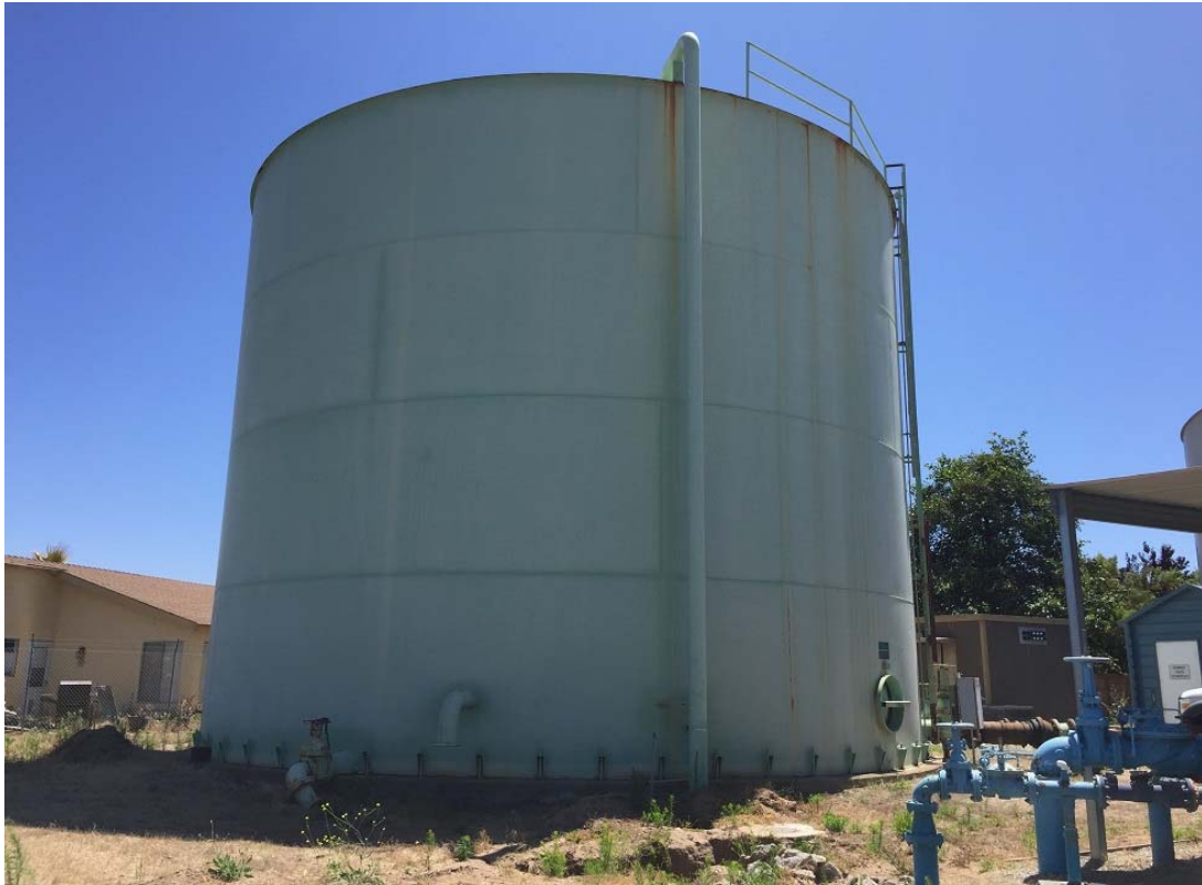
Overall view of the tank.
