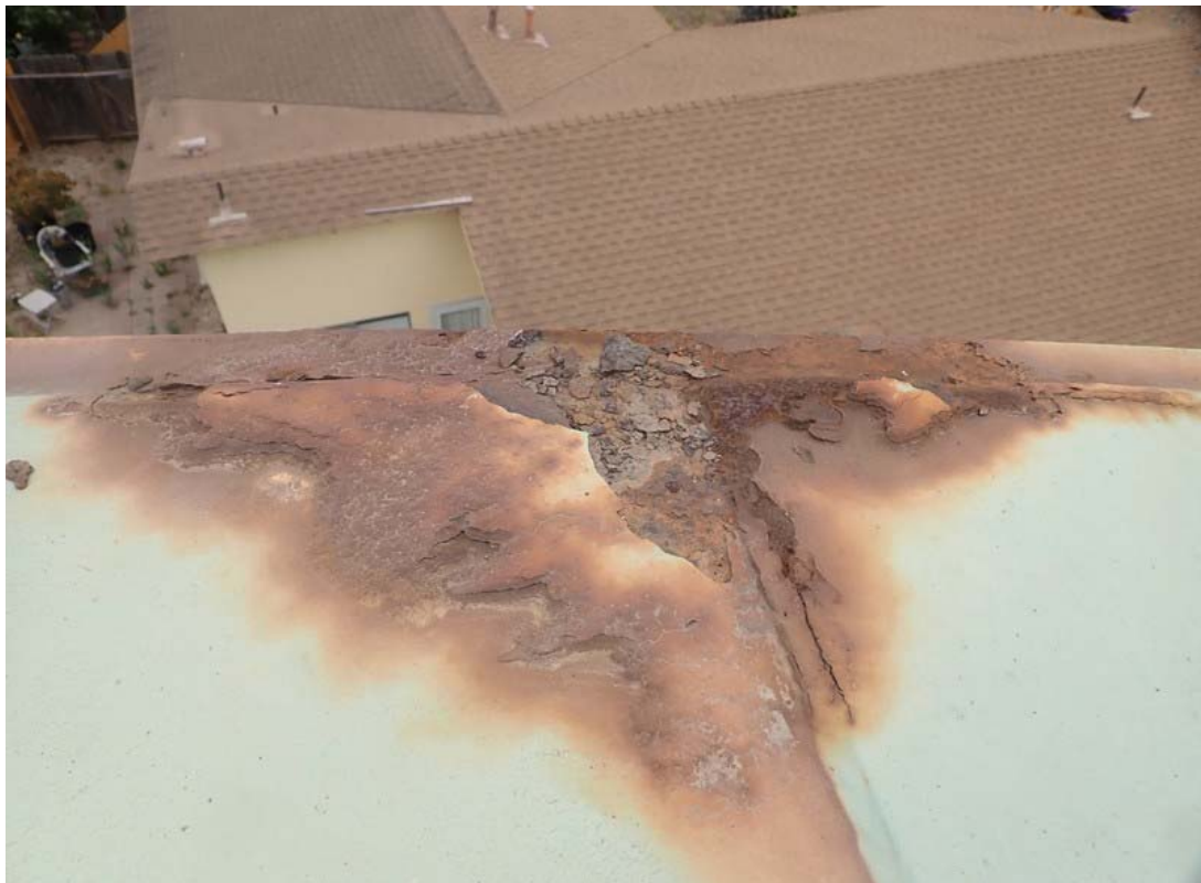
This is an addition view of a typical corroded area on the tank roof.
