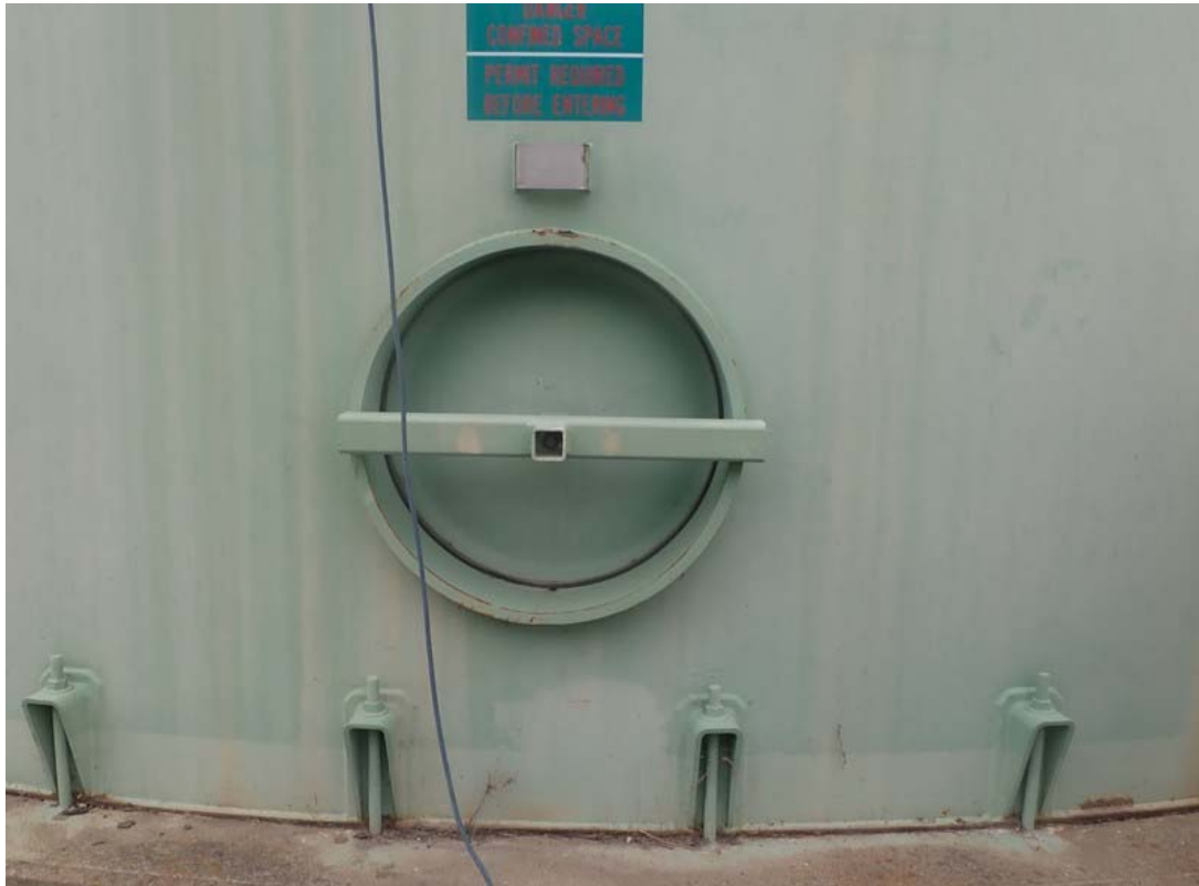
Exterior view of the manway.
