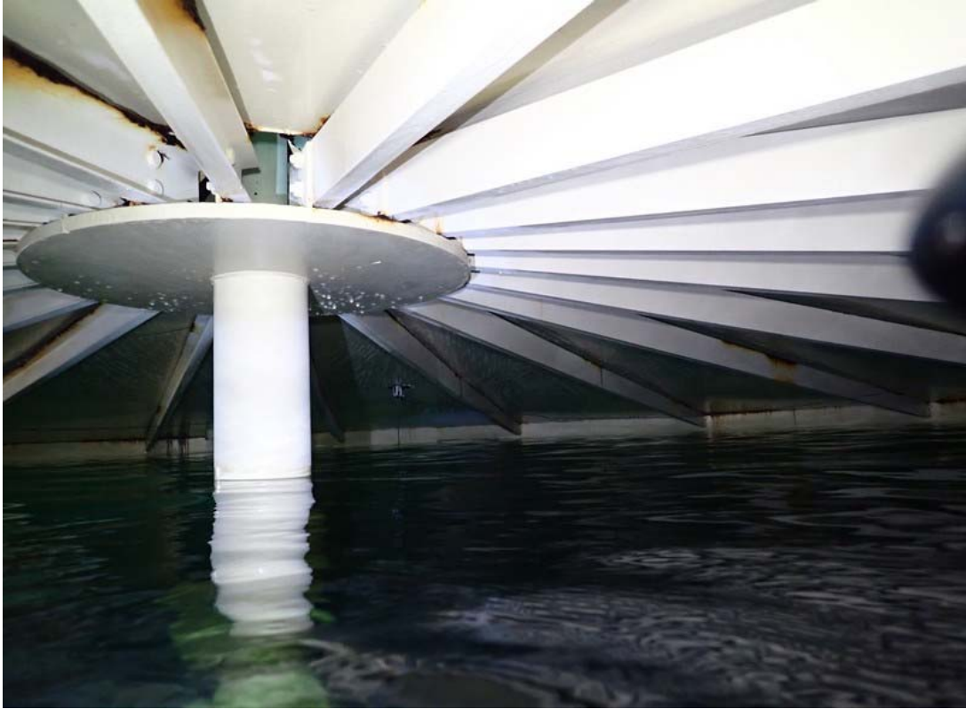
Upper center column, rafters and roof plate.
