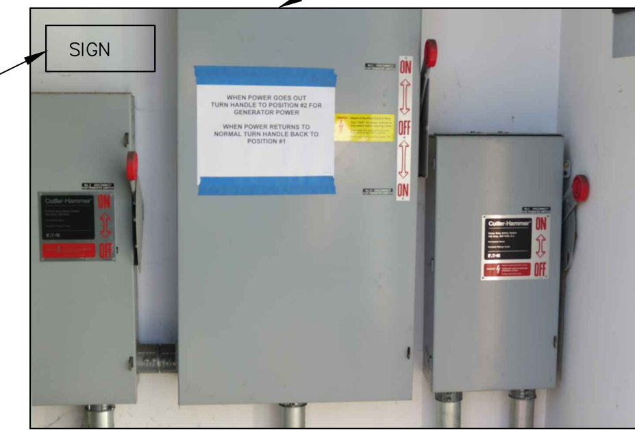
SHERIFF SUBSTATION AUTOMATIC TRANSFER SWITCH
